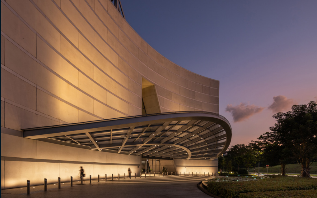
Surbana Jurong Campus, Singapore The recessed luminaires installed in the inner roof of the main entrance are harmoniously integrated into the architectural concept. Lighting design: Nipek Pte. Ltd. Photography: Finnbarr Fallon
